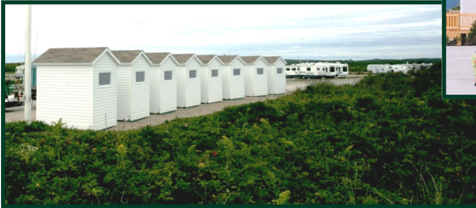
Charlestown Breachway, Charlestown, RI
